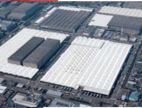
Nisson Building—After coating
