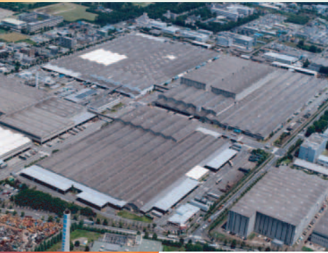
Nisson Building—Before coating
